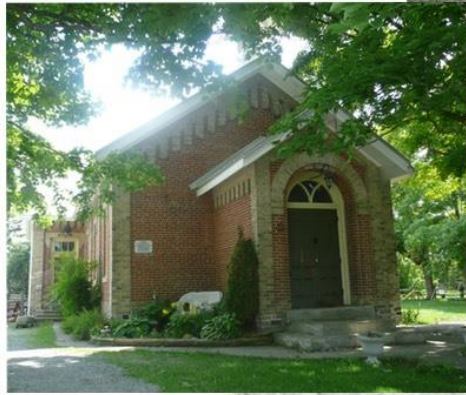
SS #1 Eldon Lorneville. The restored school is still surrounded by maple trees planted in some long-past arbour day.
